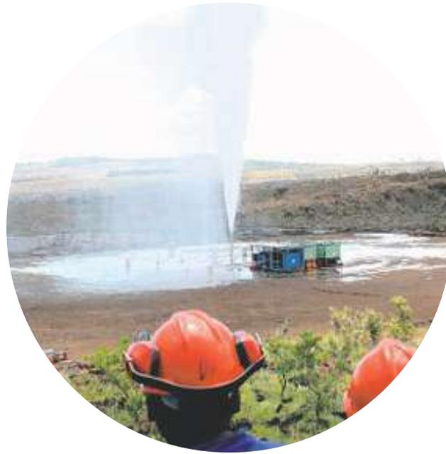
The wells will be drilled to the expedient depths about 3000 m for access of geothermal emanations (steam and water). Two operative geothermal drilling rigs need 1200 000 m<sup>3</sup> on every 60 days of drilling.
